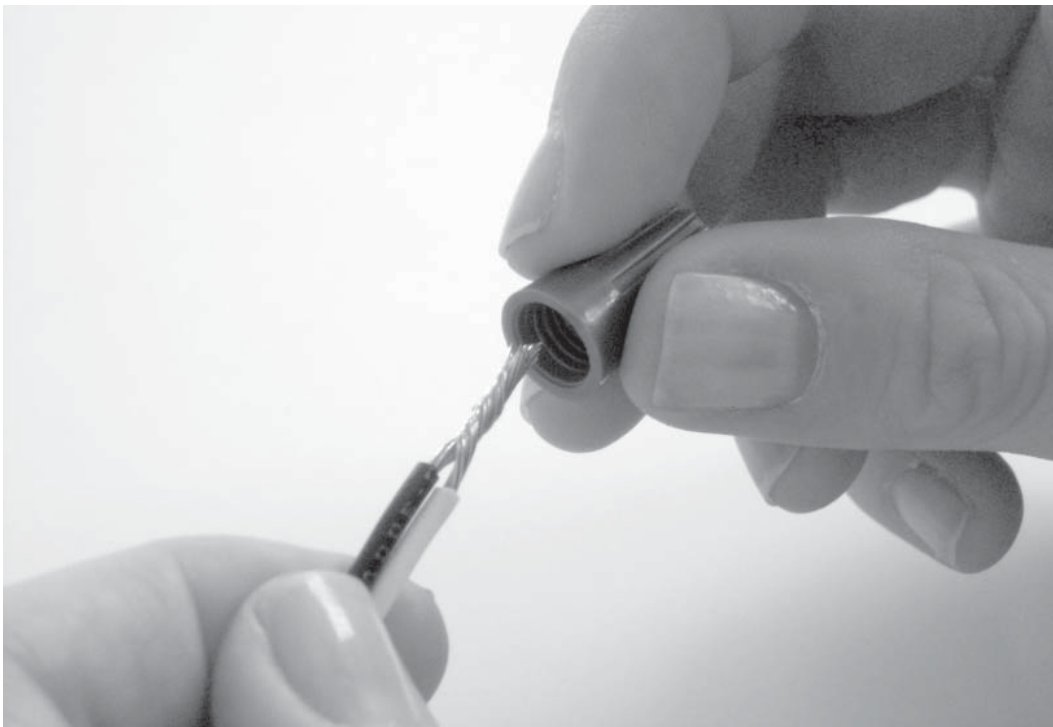
twist wire together and screw on wire nut
